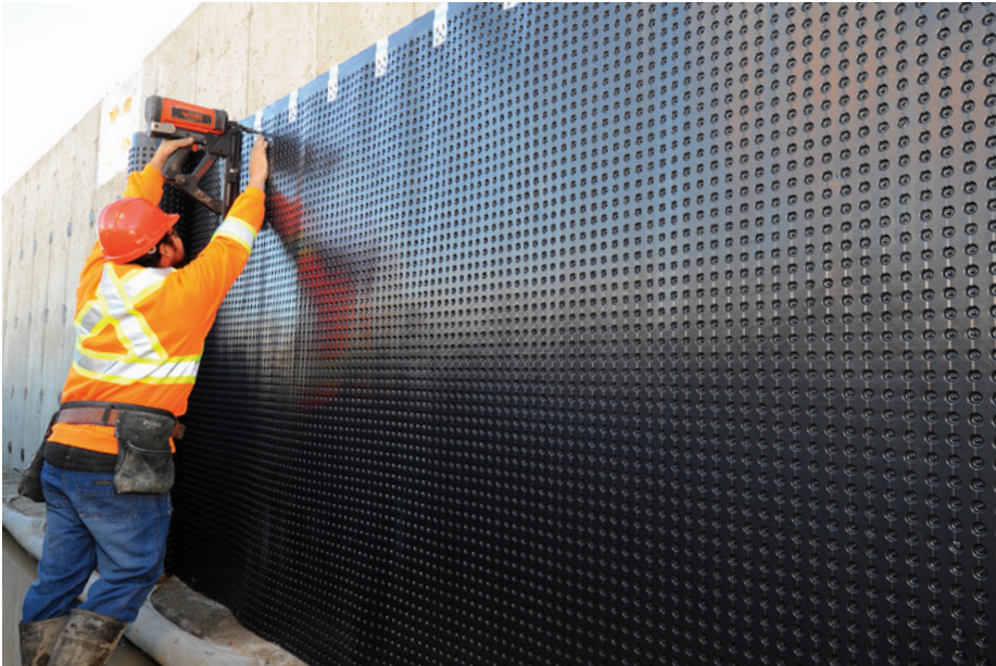
INSTALLING SPEEDCLIPS EVERY 30CM (12")
