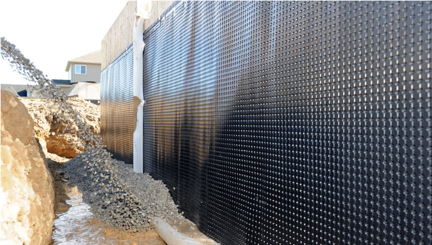
BACKFILLING OVER THE FOOTING DRAIN
